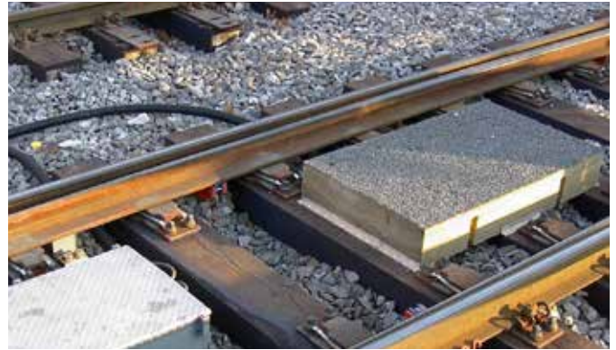
Mass detector coils
