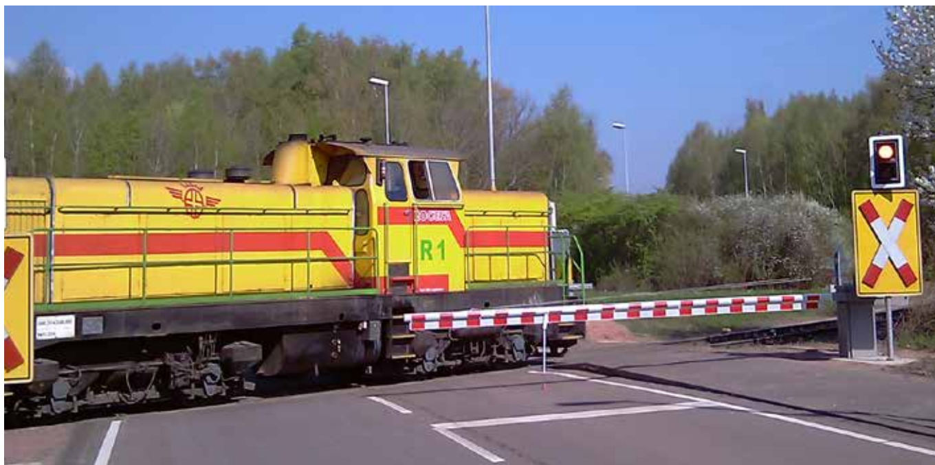
Safety installations for level crossings on industrial railways and factory sidings
