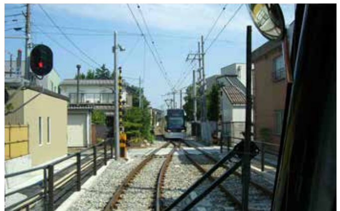
Single-line track safety devices
