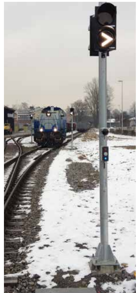
Signal transmitters for factory sidings
