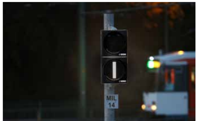
The day/night switchover generates less luminosity as daylight fades
