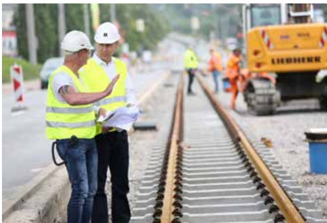
Construction management and project monitoring
