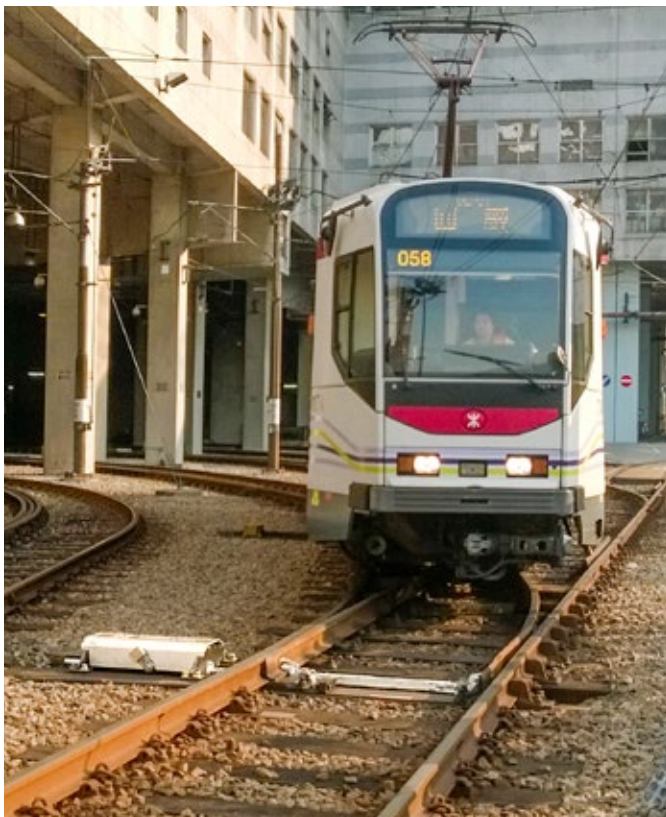
Manual point machine in the depot
