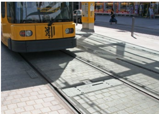
Manual point machine in the line network
